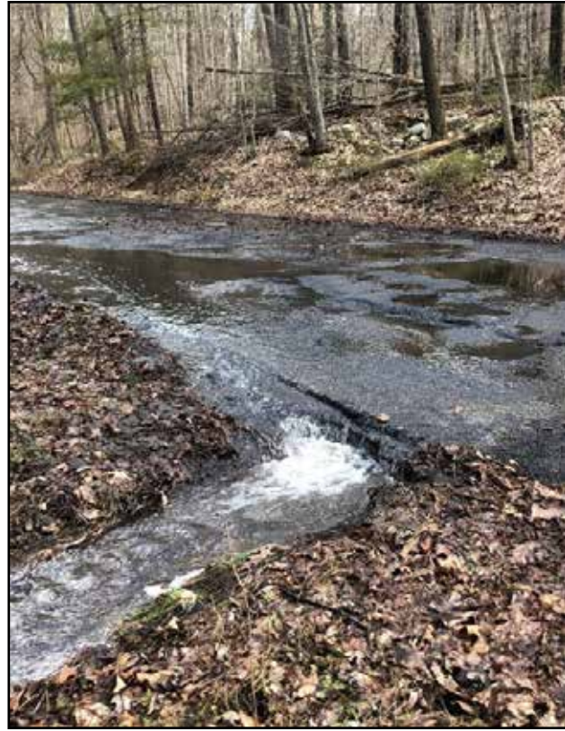
Old Mine Road riddled with potholes that are filled with water. The water is overflowing and running off the road. Photo credit: C. Palazzolo
